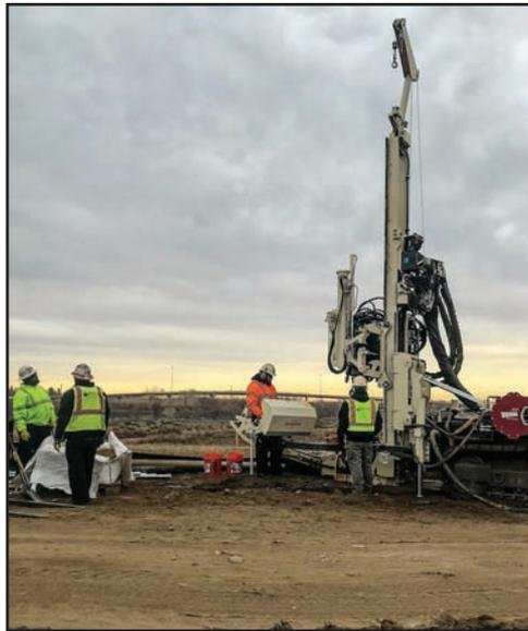
*TerraFirma utilized the Geoprobe 8150LS, operated by MW Drilling, to perform sonic drilling to reach bedrock approximately 12-17 feet belowground.*
